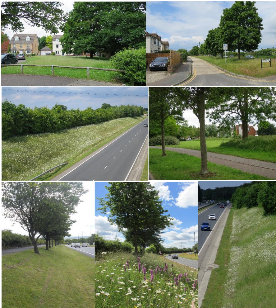
Examples of maintenance on roadside verges
